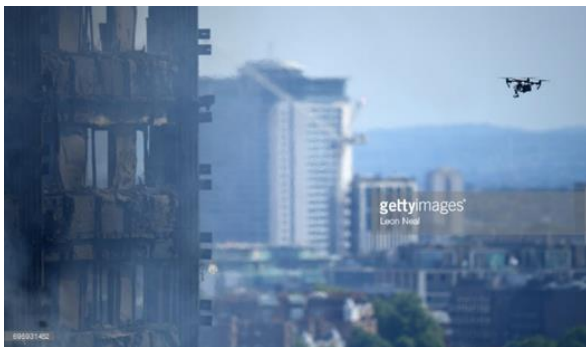
Figure 1 DJI Inspire being used to search the top floors of Grenfell Tower once the fire was extinguished.
