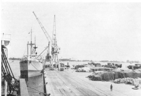
Fig.3. The container berth at Apapa (Lagos) in 1969
