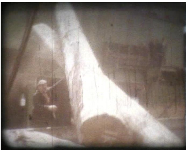
Note lack of safety hats, hi-vis jackets etc.
