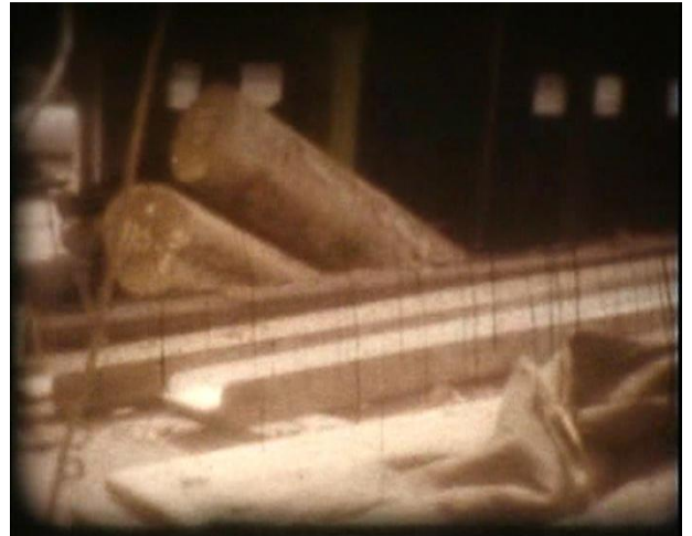
Note deck cluttered with hatch beams & boards
